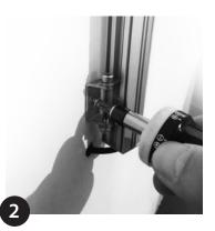
Fix bracket with suitable screws.
